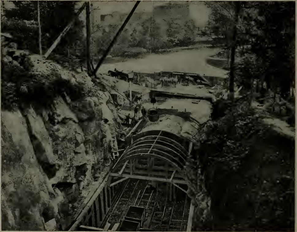
Open Cut Subway Construction in Central Park, Lenox Avenue Branch.
